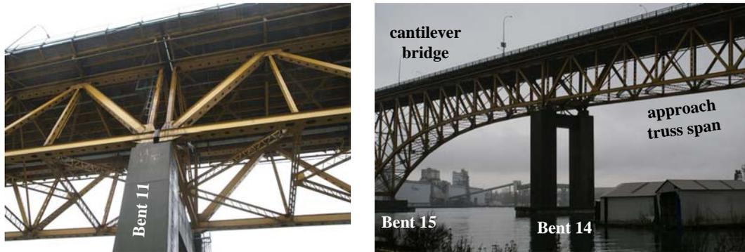
a) Deck floor and steel warren trusses
