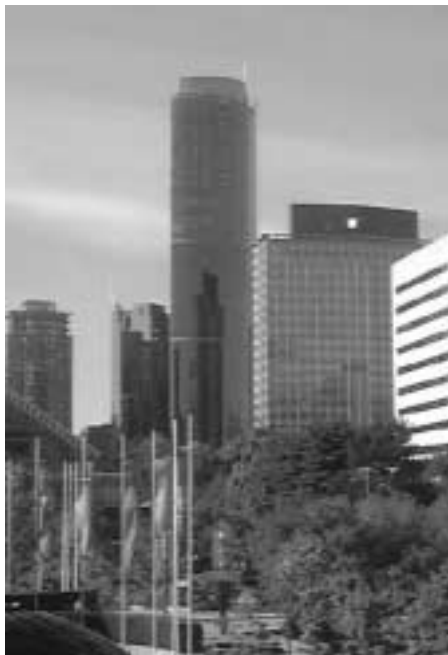
Fig. 1: North face of the One Wall Centre
