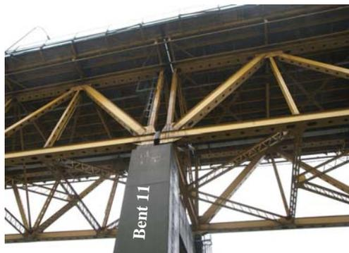
a) Deck floor and steel warren trusses
